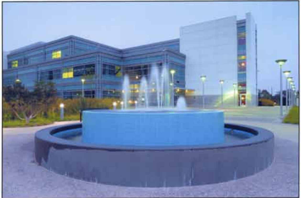
The Genentech campus in Oceanside won the ISPE 2007 Facility of the Year award for utilizing innovative technologies to improve product quality and reduce cost of production.
