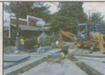
Utility lines in Julian almost done
