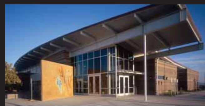
Department of Motor Vehicles, San Ysidro Field Office Architectural Firm: Roesling Nakamura Terada Architects, Inc. Photo By: Kevin Walsh, Kevin Walsh Photography
