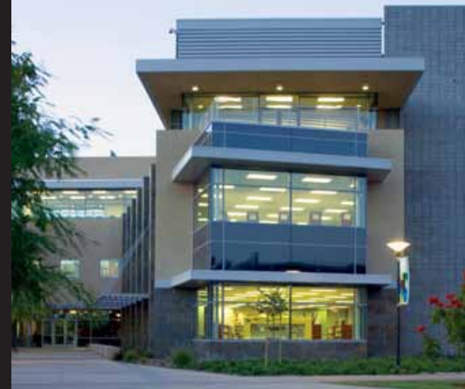
La Jolla Country Day School Library Academic Center Architectural Firm: Ferguson Pape Baldwin Architects Photo By: Frank Domin, Domin Photography
